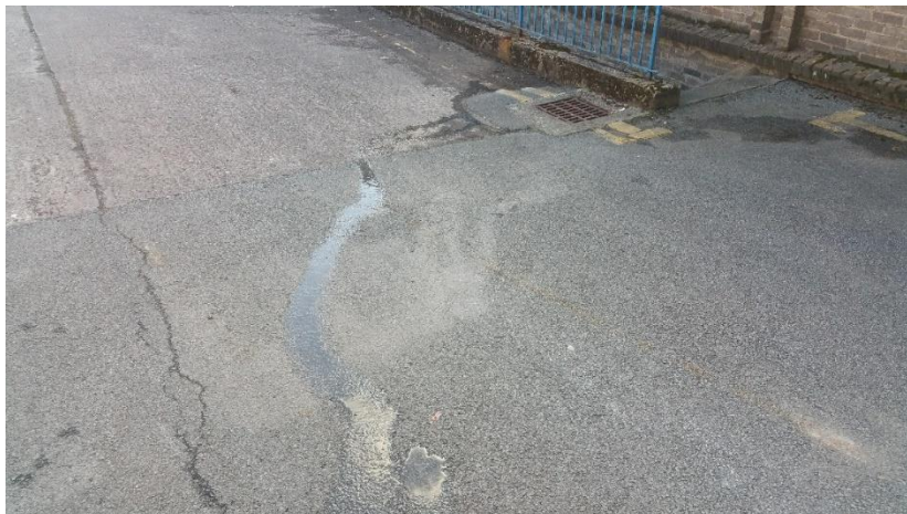
Figure 36: Photographs of first carpark experiment attempt, showing drainage towards water drain
